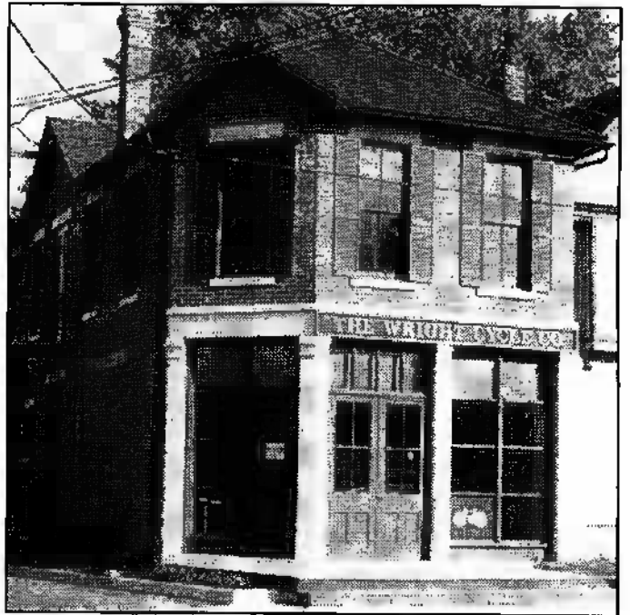
The Wright Brothers Bicycle Shop at 22 South Williams Street in 1991 after restoration by Aviation Trail, Inc.
